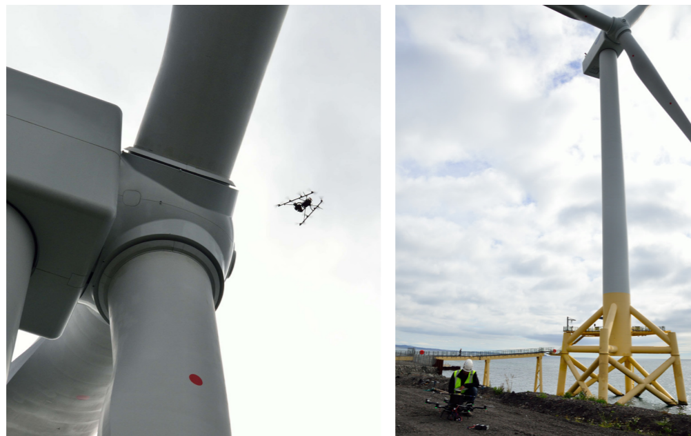
Figure 11: ORE Catapult's UAV blade inspection at Levenmouth Demonstration Turbine in Scotland.
